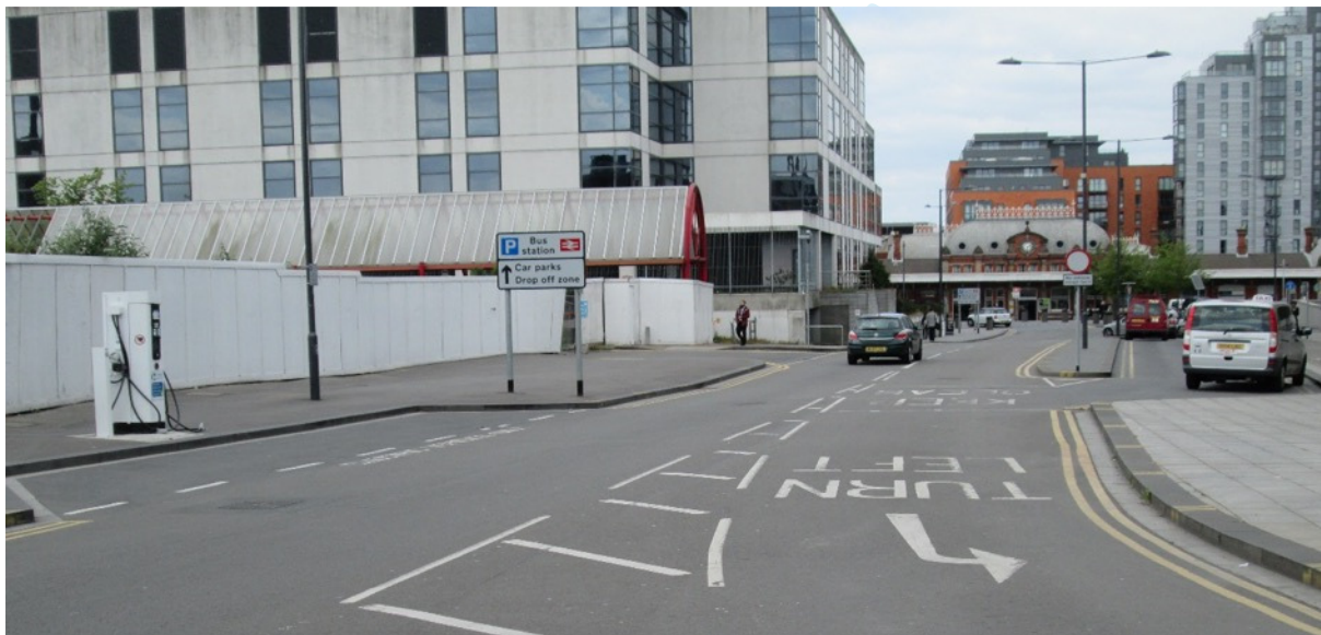
Rapid charging unit on Brunel Way with Slough Station Taxi Rank opposite
